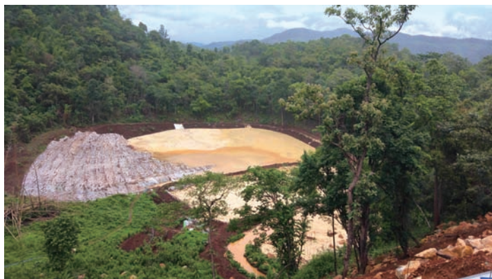
The tailings storage dam of the Aung Jiuja Mine has adopted sufficient anti-seepage measures, which effectively prevent the leakage of tailings.
